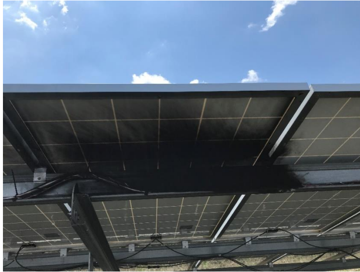
Figure 13 Failed wiring
